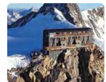
Monte Rosa Mountain Hut Margherita
